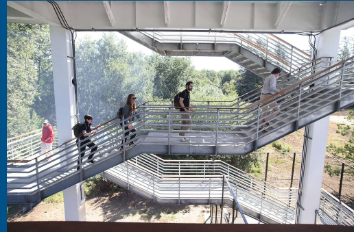
Members of the Washington state Department of Natural Resources and Emergency Management Division walk up the stairs of the vertical evacuation structure.
