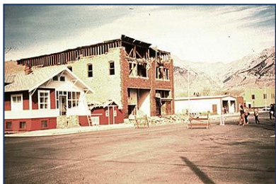
Unreinforced masonry buildings are susceptible to shaking and create debris.
