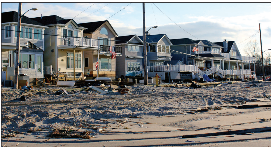
Figure 1: Homes on small, tightly spaced lots, typical throughout coastal New York and New Jersey, present access and construction challenges when being transitioned to a raised pile foundation (Rockaway, NY).
