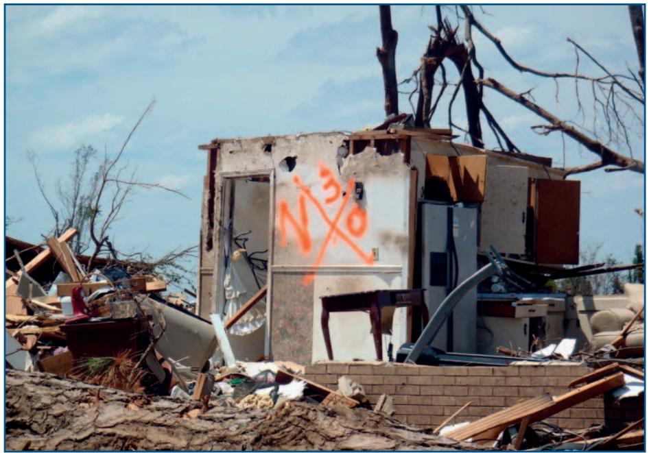
View of remnants of an interior room of a house that survived a strong tornado (Tuscaloosa, AL).
