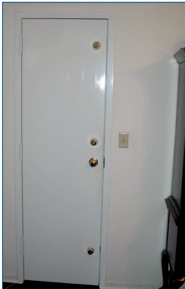
Photograph of safe room door with three deadbolts and three hinges.
