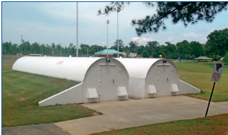
View of a partially below-grade community safe room at a manufactured home community (Brookwood, AL).
