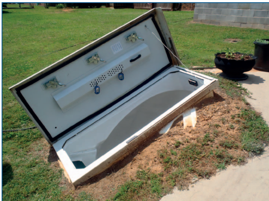
View of a pre-fabricated safe room that serves a few manufactured homes (Tuscaloosa, AL).
