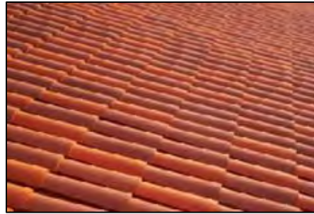
Clay tile roof
