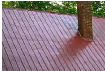
Standing seam metal roof
