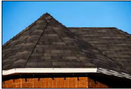
Asphalt shingle roof
