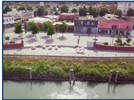
Figure 1: The new floodwall is an integral part of the downtown promenade, providing flood protection and public recreation space.
