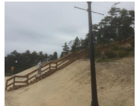
South stairway to Safe Haven
