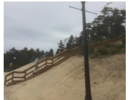
South stairway to Safe Haven
